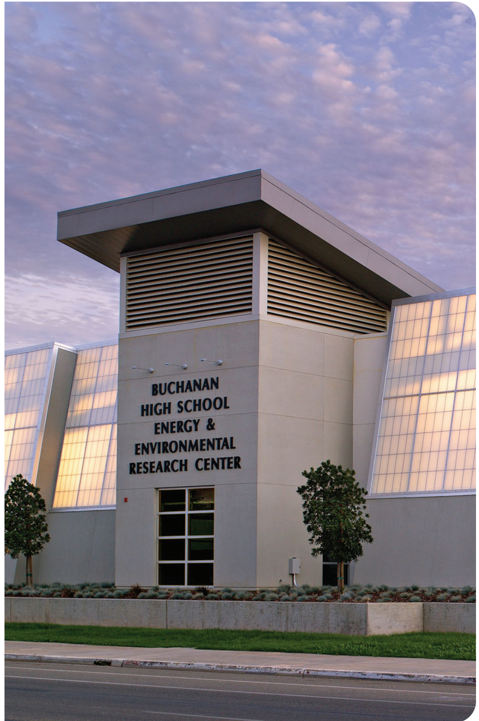
The Buchanan Center, featuring Solarban® 70 glass by Vitro Architectural Glass (formerly PPG glass), earned a 2011 Excellence in Design Award from ED+C magazine in the educational category.
